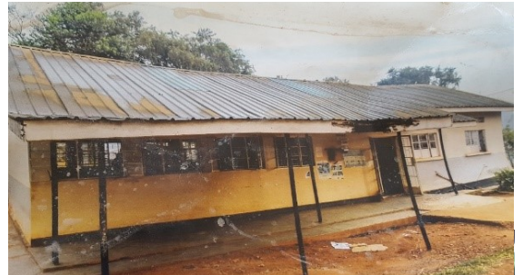
A facility pre-makeover
